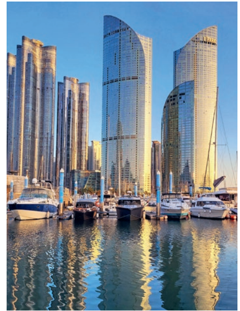
High-Rise-Buildings in Busan
